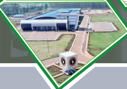
NEC CONSTRUCTION WORKS AND ENGINEERING
