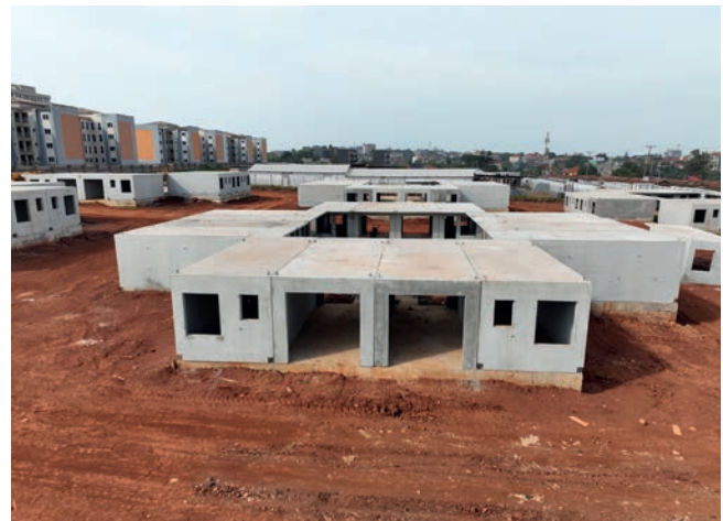
The Naguru Apartments Phase II
