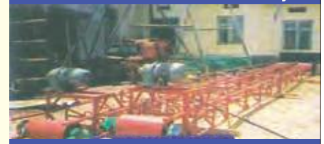
Fabrication of Conveyors,
