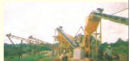
Fabrication and Installation of Quarry
