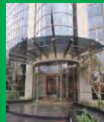
Glass Canopy and Skylights
