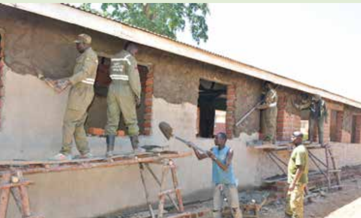
UPDF Engineers Brigade experts renovating acounciling building at Kitgum main Hospital.
