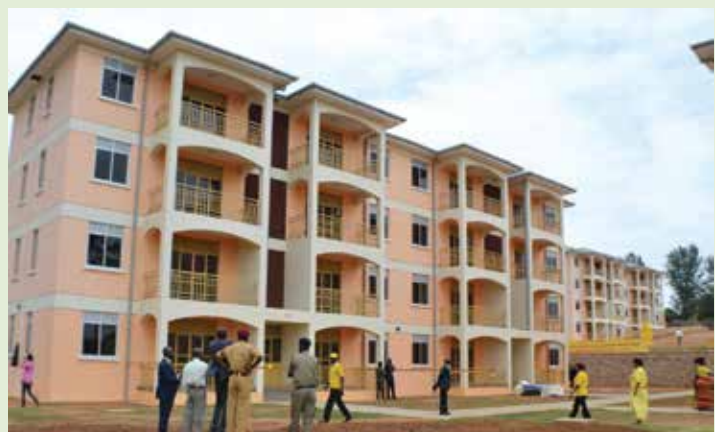
UPDF Engineering Brigade built Masaka flats.
