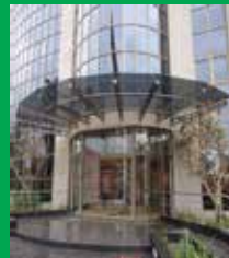
Glass Canopy and Skylights
