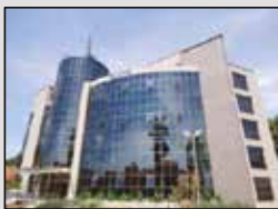
Curtain Wall & Structural Glazing
