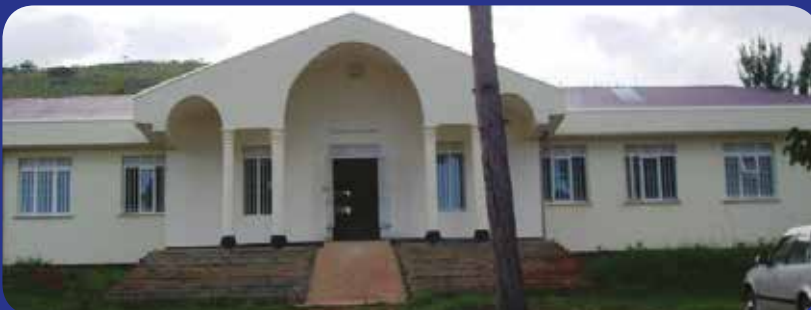
Ibanda District Local Government Water Office Block
